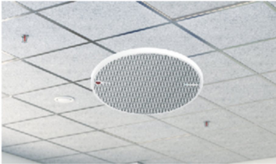
1 Flush installation in the ceiling grid
